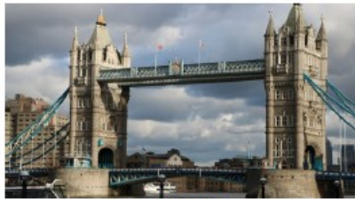
Tower Bridge London, England
